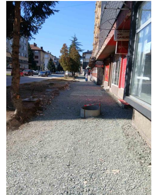
Works in progress, Sept 2026
